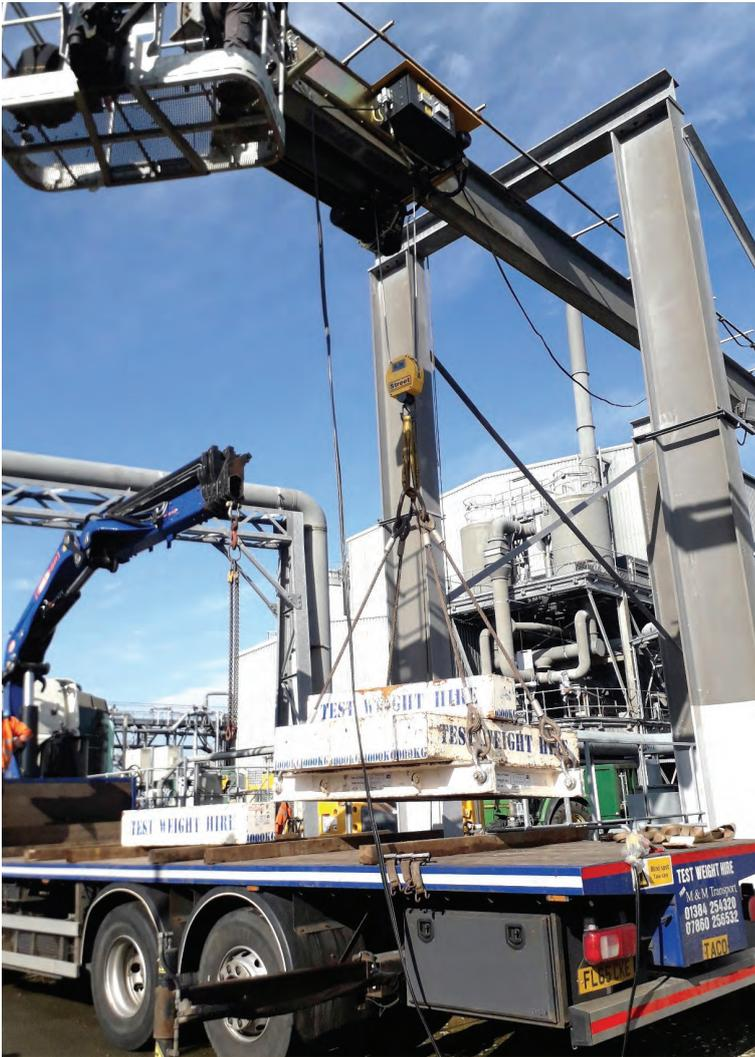
Street Cranexpress carrying out the proof load test of the newly installed Street hoist
